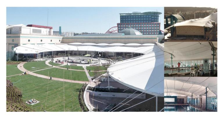
The roof of the Colombo Shopping Centre was built over an already existing swimming pool, with a covered surface area of 3,100m2. The main condition required in the design was simple dismantling of the structure.
